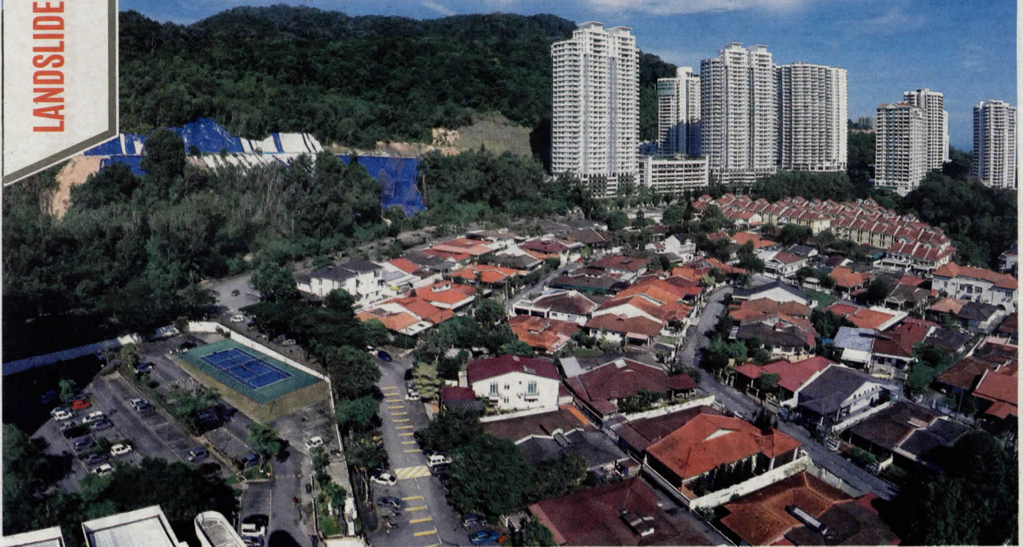
Highrise housing in Tanjung Bungah. Habibah says landslides are prone in the area because the soil composition is largely made of rocks that are being eroded.
