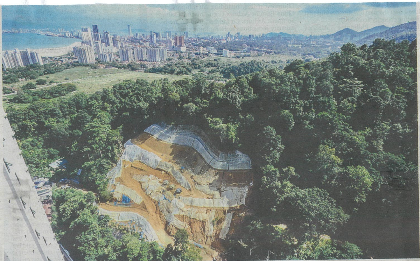
Earthworks and hill-cutting at Mount Erskine yesterday. – BBXPIX
