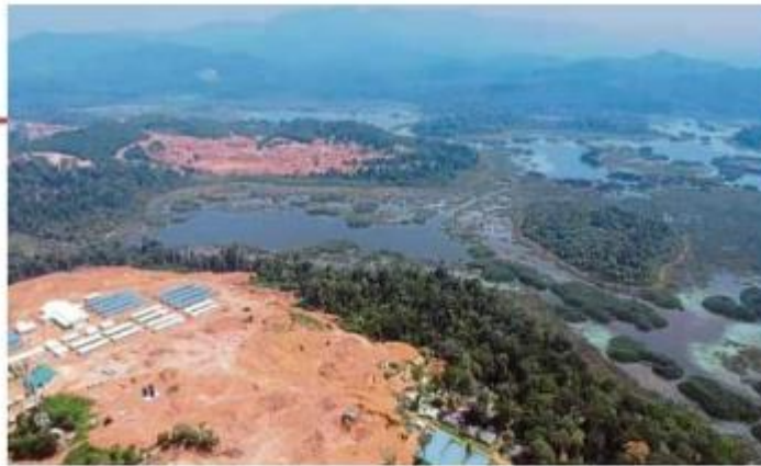
A section of hillside next to Tasik Chini in Pahang which has been cleared for logging and mining activities. PIC BY FARIZUL HAFIZ AWANG
