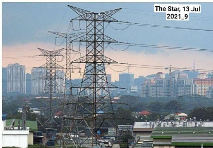
The electricity grid of the future will not be just wires and cables carrying electricity from one place to another.
