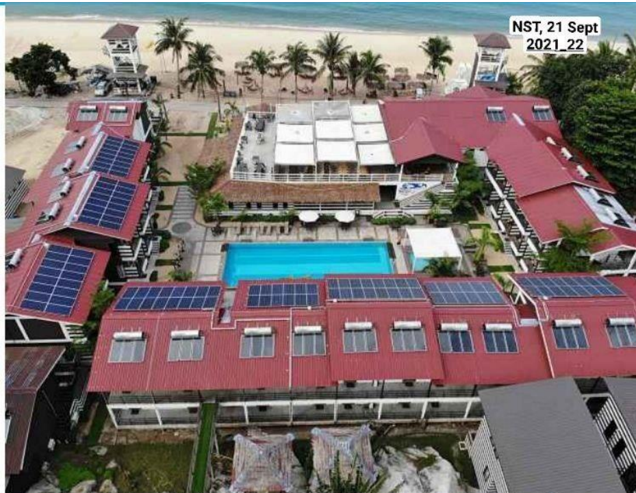
Pekat Solar Sdn Bhd's award is for the Energy Storage System at the Barat Tioman Beach Resort.
