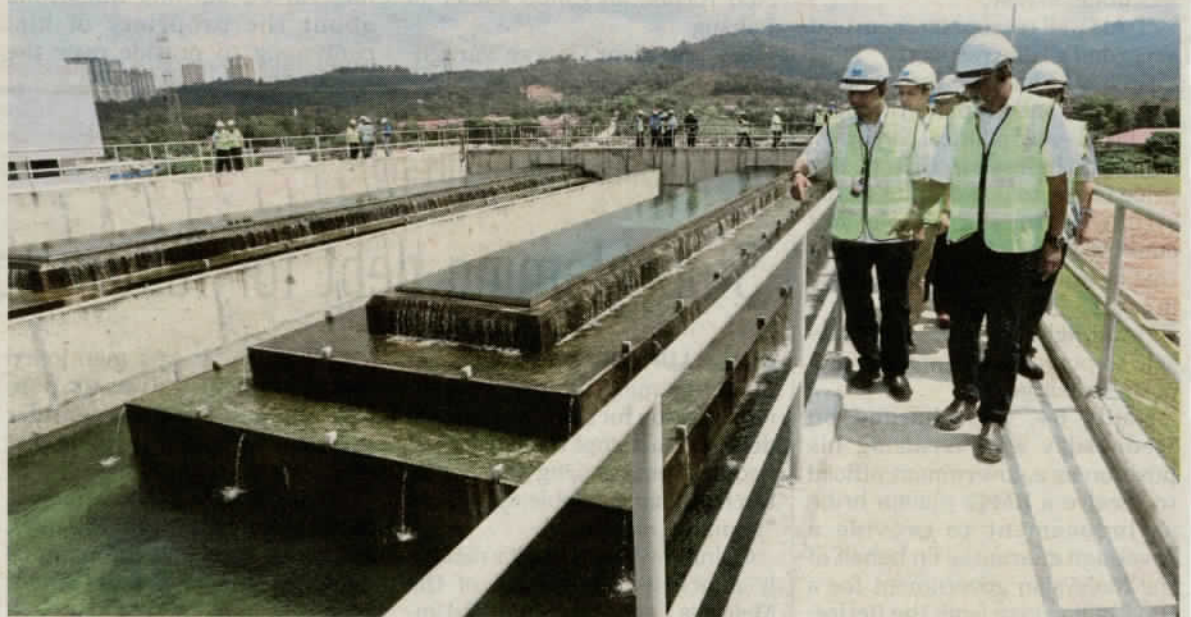
Water, Land and Natural Resources Minister Dr Xavier Jayakumar (right) at the Langat 2 Water Treatment Plant in Hulu Langat yesterday. PIC BY ZULFADHLI ZULKIFLI
