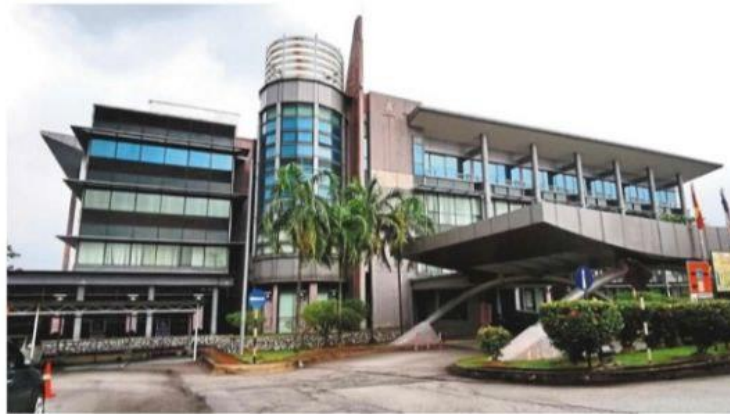
Some suggest that a manual backup system should be maintained at land offices such as this one, which is the Petaling District Government Office and Land Registry Department in Shah Alam.
