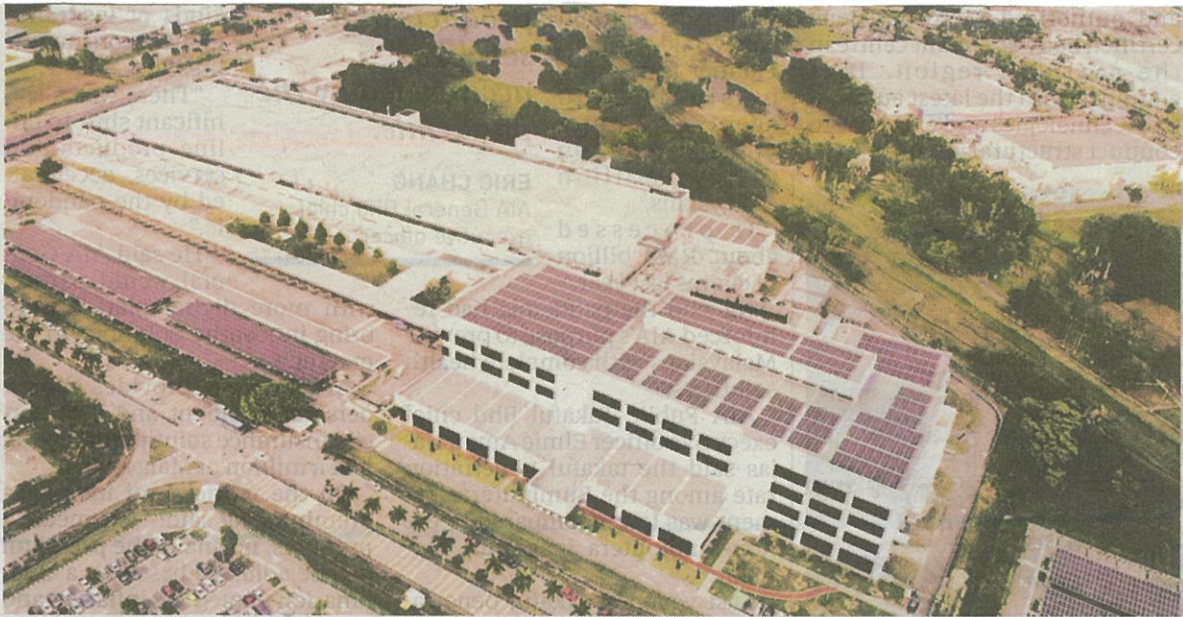
The new solar farm panels at Intel Malaysia cover an area roughly equivalent to 900 carpark spaces and an additional 50,208 sq ft on buildings' rooftops.
