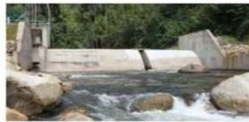
The Gunung Hydropower Sdn Bhd-Tenaga Nasional Bhd power purchase deal involves the mini-hydropower plant off Sungai Perak in Salu.
